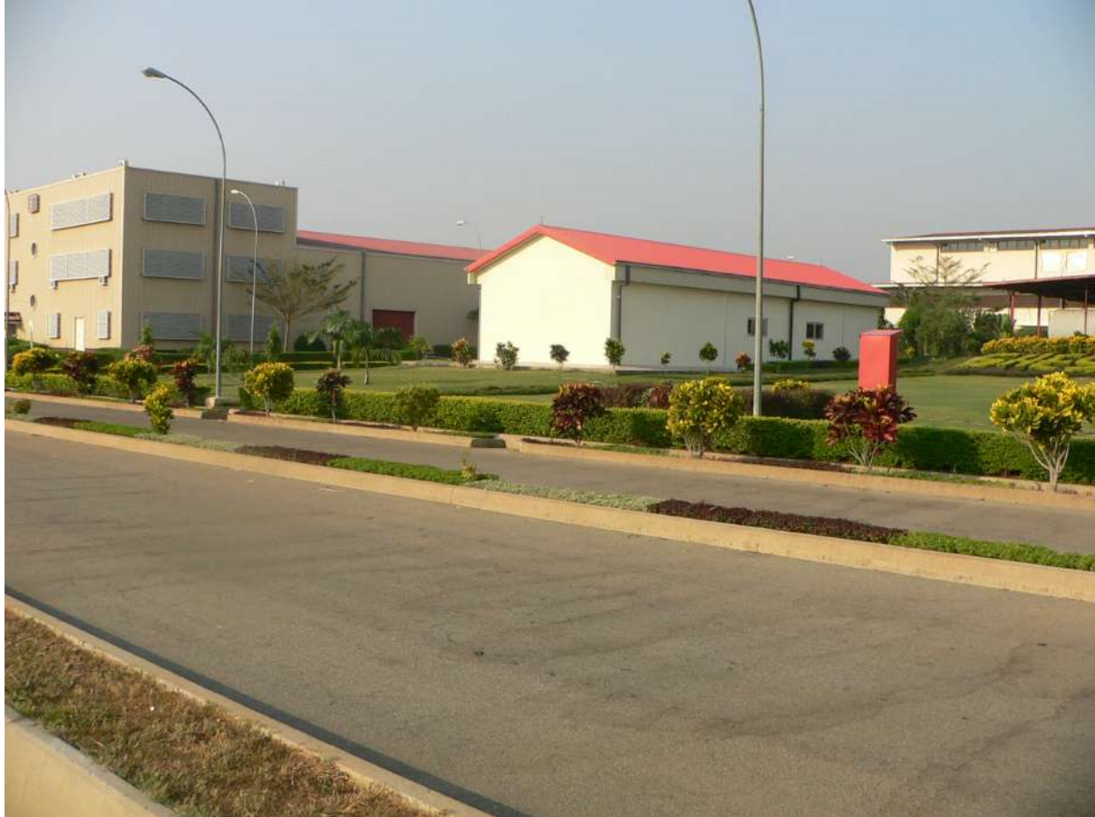
Picture showing some of the facilities of the Nuclear Technology Centre: Central Mechanical and Electrical Workshop (left); Water Treatment Plant House (middle); and Gamma Irradiation Facility Building (far right).
