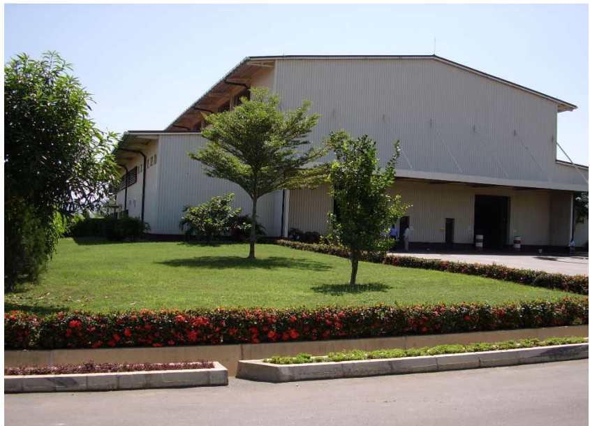
The Gamma Irradiation Facility Building
