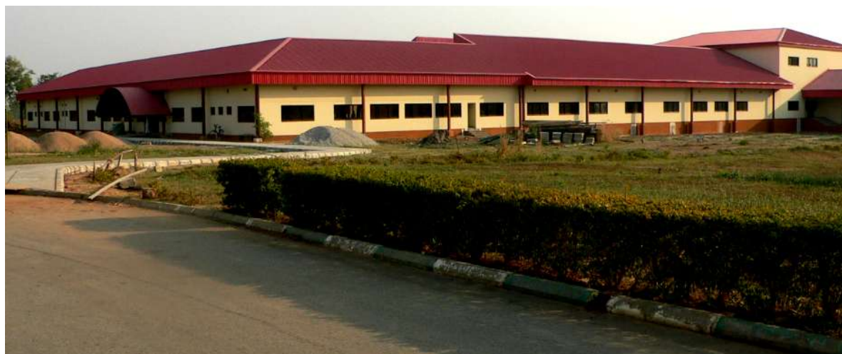
New Biotechnology Laboratory Complex under construction
